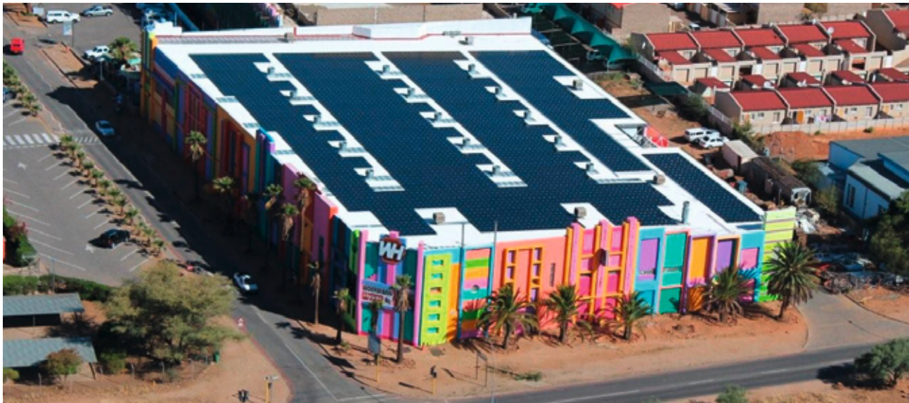
The installation on the roof of a Woermann supermarket is currently the largest PV installation in Namibia with more than 300 kWp. (Image: HopSol)
